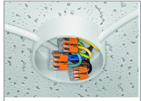
Lighting distribution in a ceiling canopy
