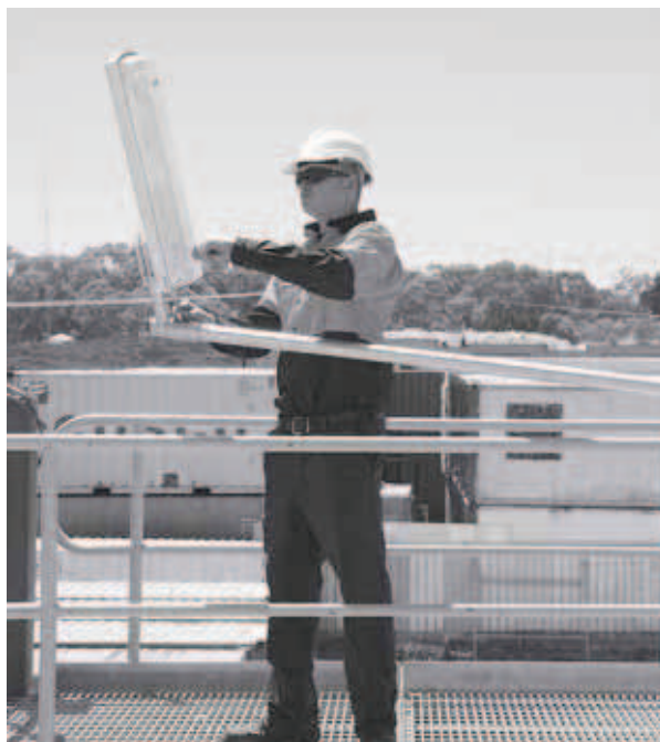
Safe and easy access to luminaire for inspection and regular maintenance
